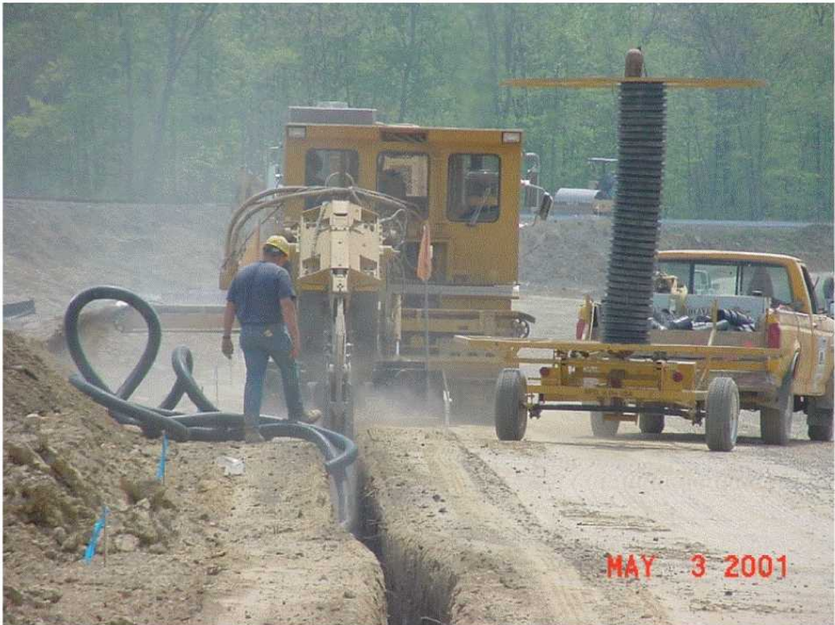
Figure 8-4. Underdrain installation ( photo courtesy of Ohio DOT ).
