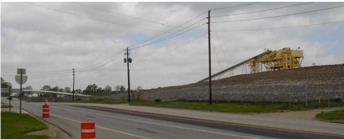
Figure 8-10. Earth-moving conveyor system ( Atlanta Airport – 5 th Runway Embankment Placement ).
