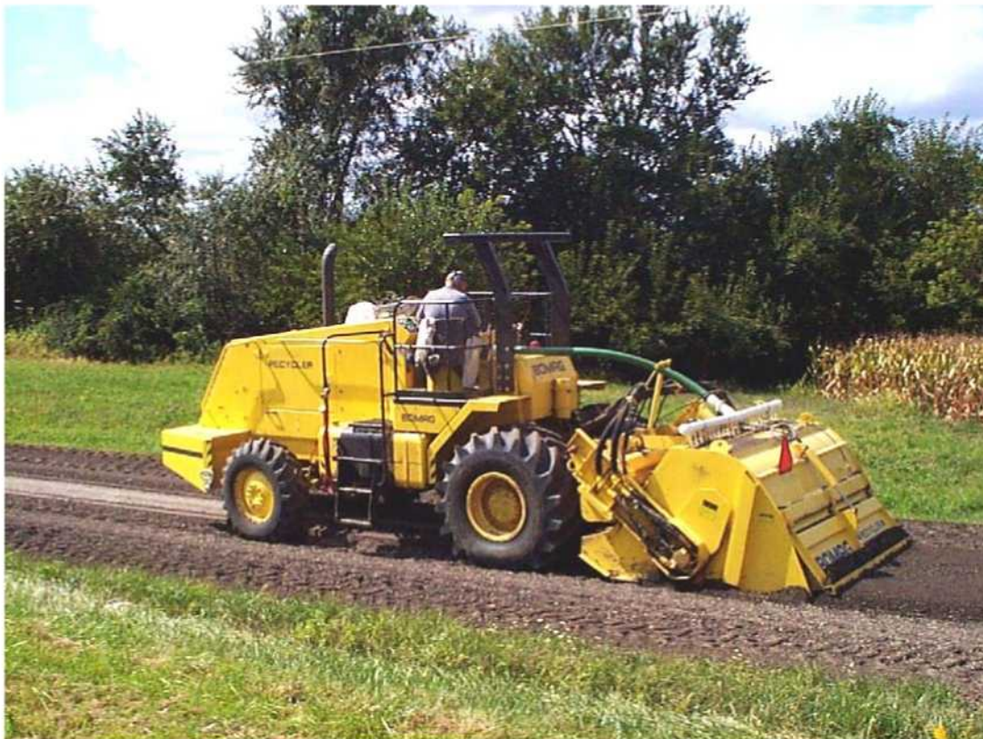
Figure 8-16. Roadway stabilizer/mixer (photo courtesy of Bomag).
